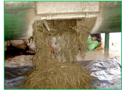
Mixing wood wool, cement and water
